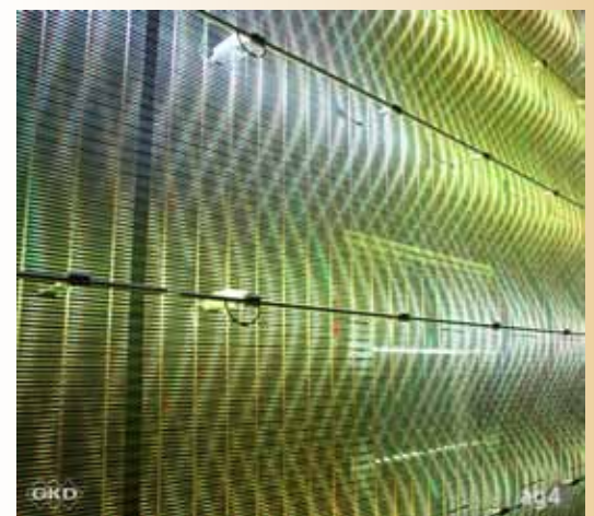
The stainless steel mesh surface of this Illumes® installation in Torce, France, shines with reflected sunlight during the day and glows with an ever-changing display of light and color at night.
