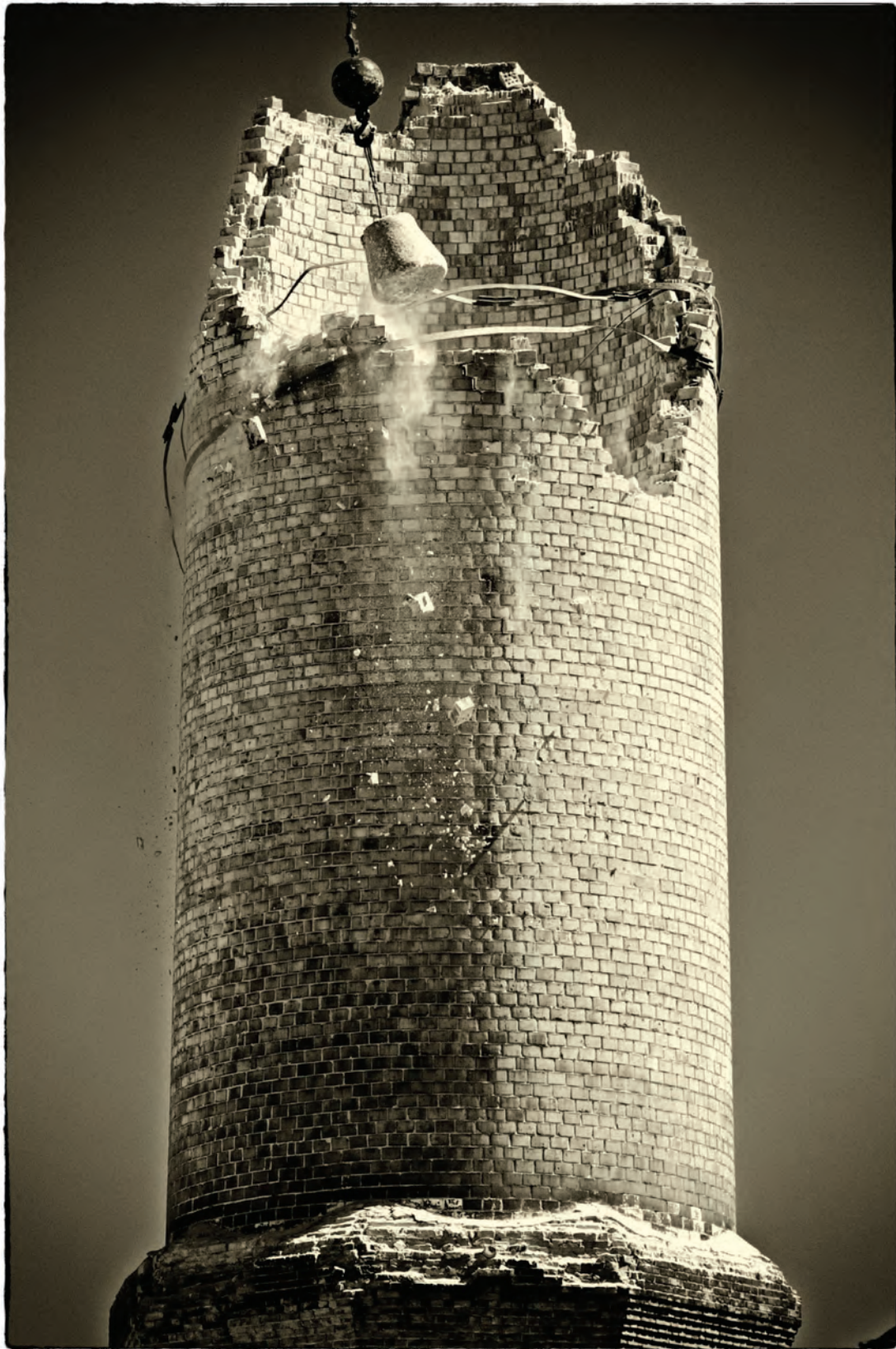
The demolition continues, American Thread Mills Bldg. No. 2 smokestack, Willimantic, Conn.
