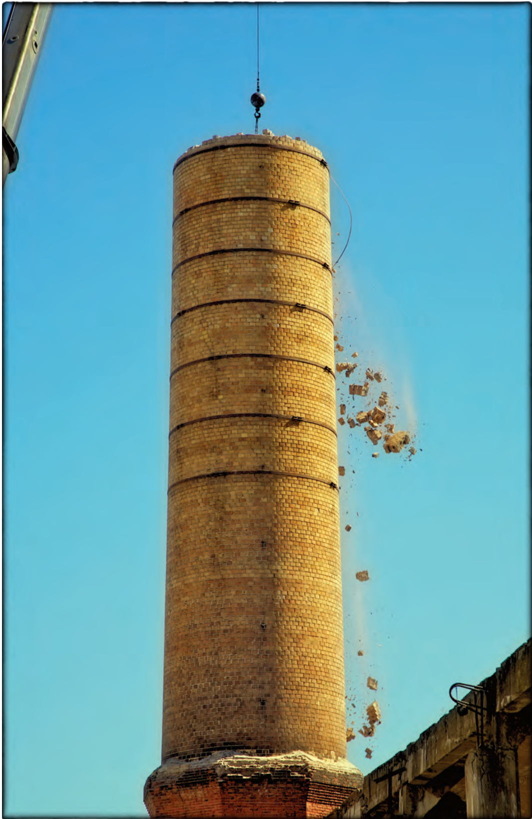
The demolition begins, American Thread Mills Bldg. No. 2 smokestack, Willimantic, Conn.
