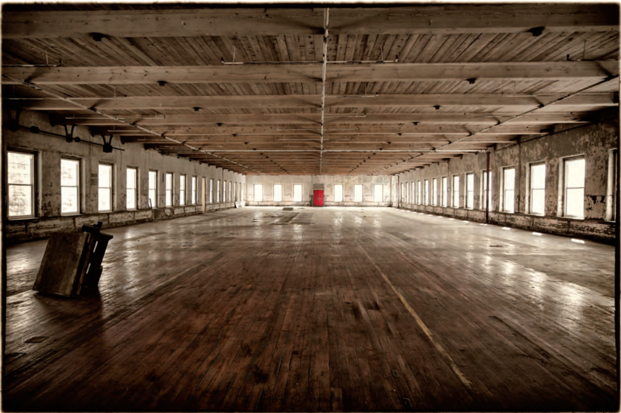
Top floor, American Thread Mills Bldg. No. 2, Willimantic, Conn.
