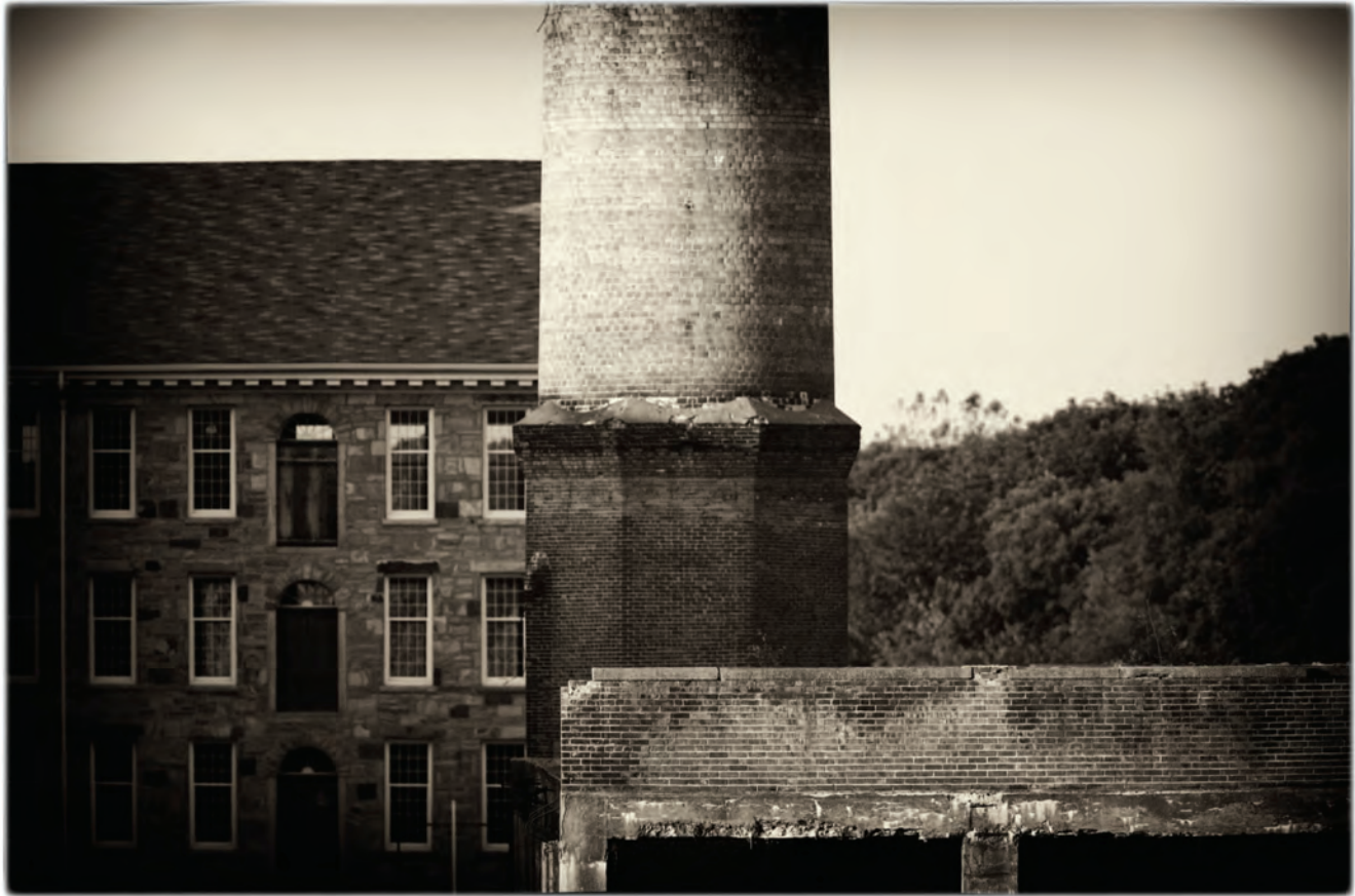
American Thread Mills Bldg. No. 2 and its smokestack, Willimantic, Conn.
