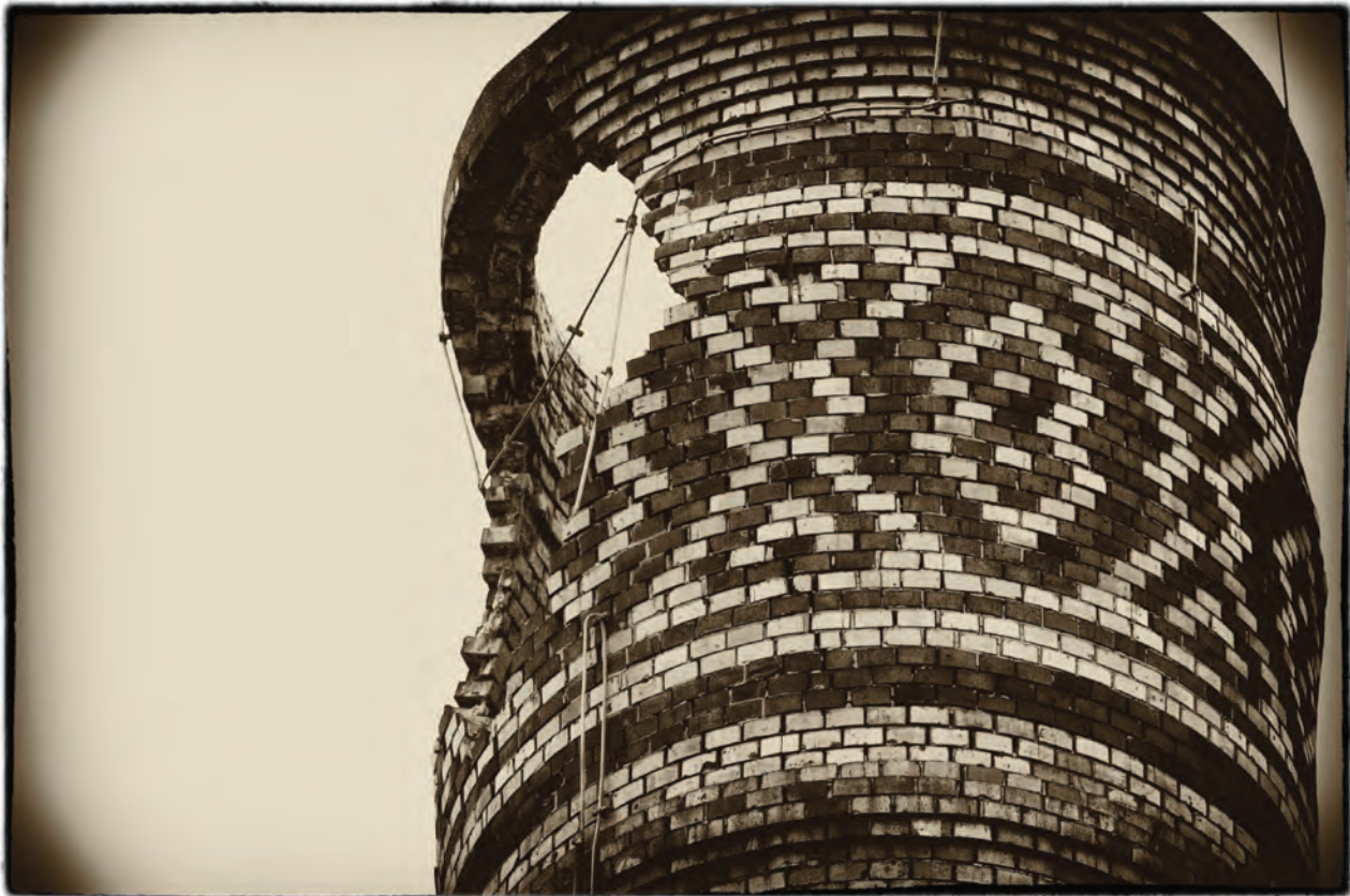
Close view of winter storm damage, American Thread Mills smokestack, Willimantic, Conn.
