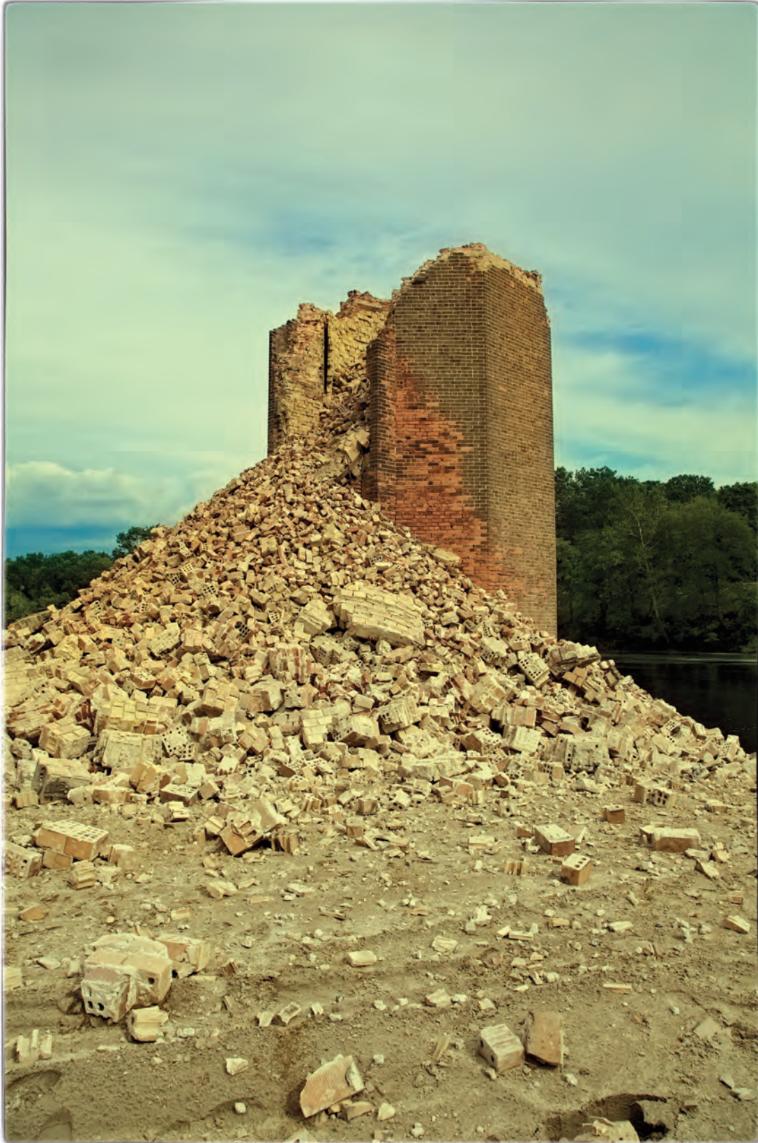
The demolition completed, American Thread Mills Bldg. No. 2 smokestack, Willimantic, Conn.
